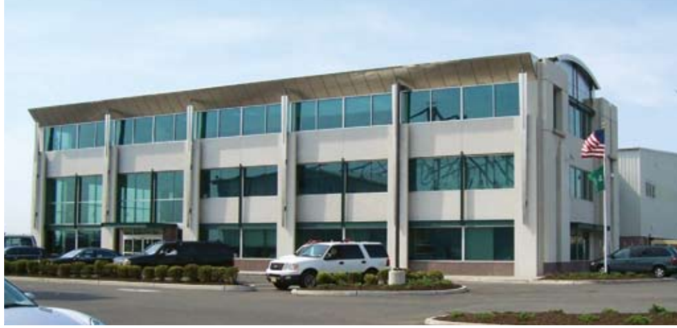
The terminal's ornate, architectural use of precast includes "T"-shaped columns used as accent pieces on the structure's north side. Photo: David Zugale.
