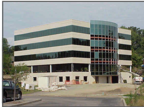
Franklin Park Corporate Office Building during the precast erection phase of construction.
