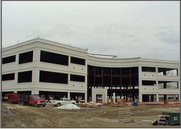
Landerhaven II Office Building during the precast erection phase of construction.
