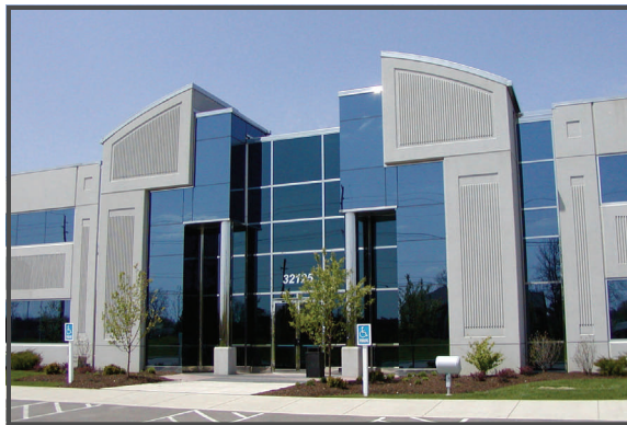
Exterior views of the Solon Marquis Office Building.
