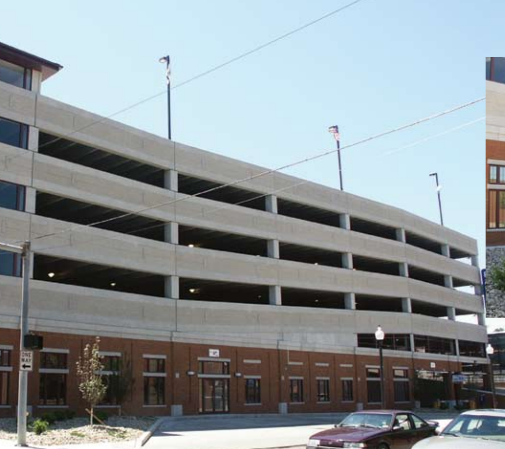
The new Parkersburg, W. Va., intermodal/mixed-use parking facility was produced on a design-build contract. It features an all-precast concrete structural system that helped meet the deadline and budget.
